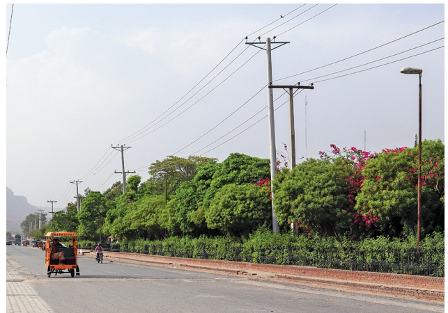
Extension of the footpath and walkway from Khewra to Pind Dadan Khan
